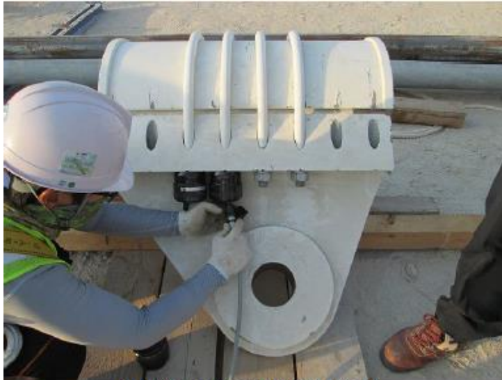
Bolt Tensioner Fit up Test
