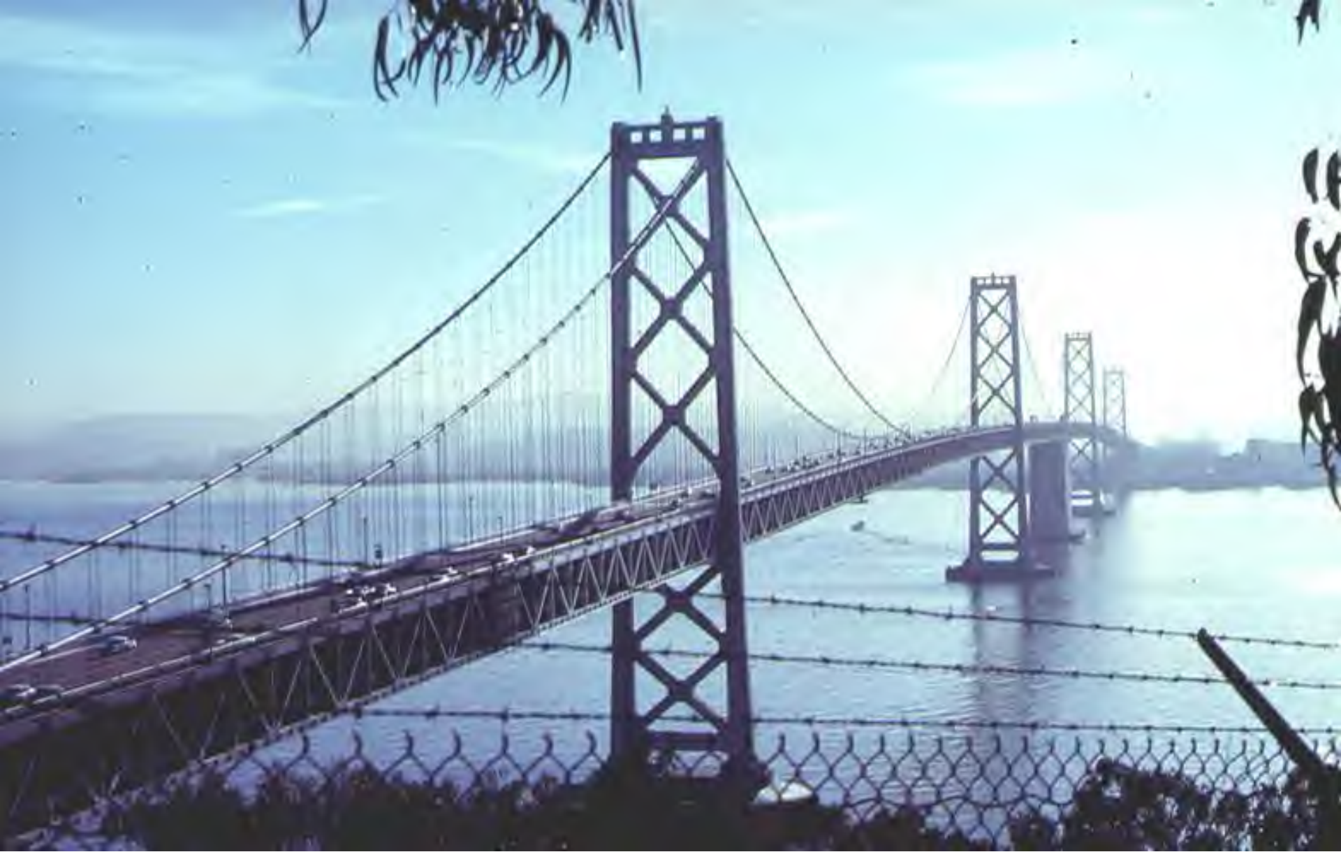
San Francisco-Oakland Bay Bridge (1936)
