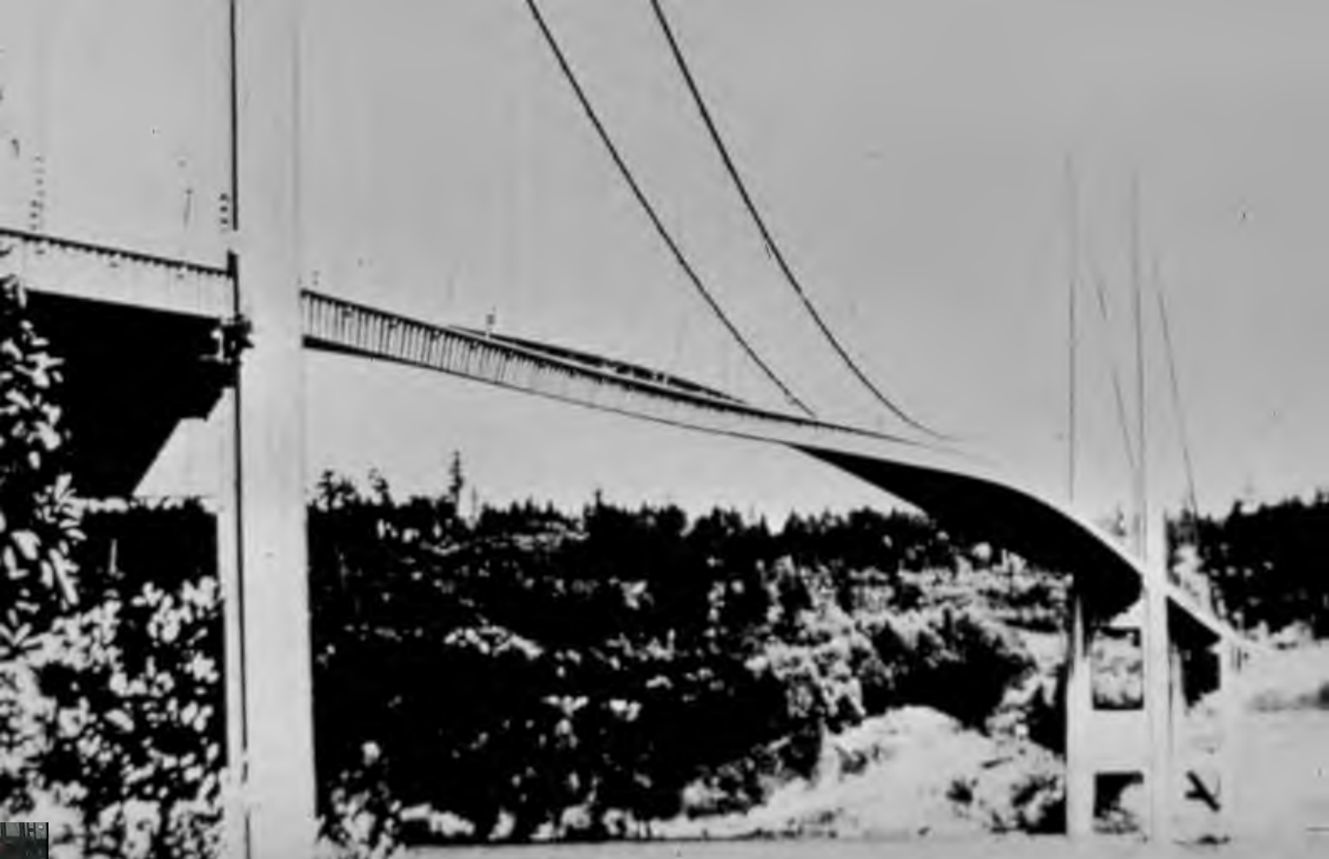
Tacoma Narrows Bridge (1940) 855m
