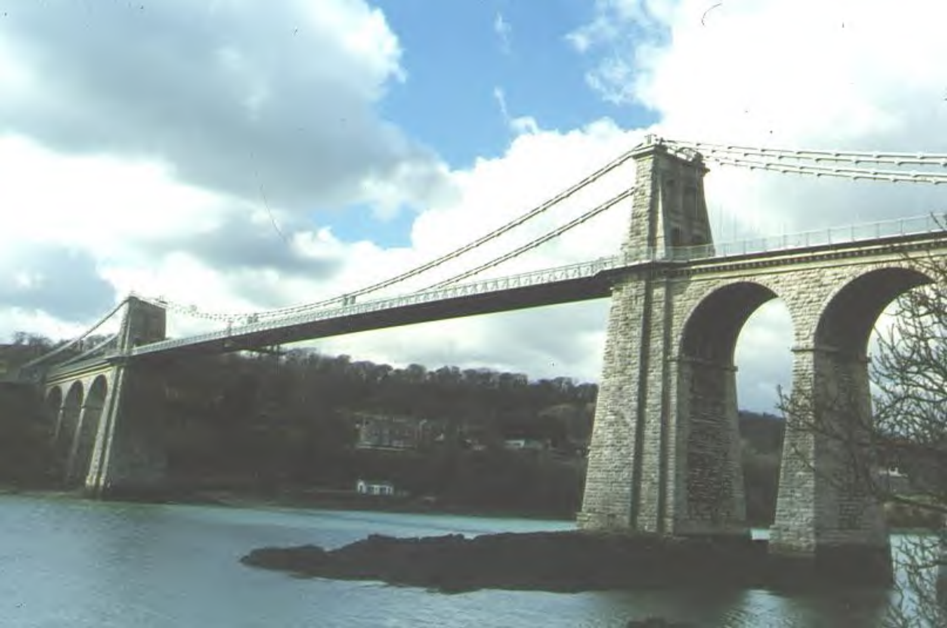
Menai Bridge 1826 (British) 176 m
